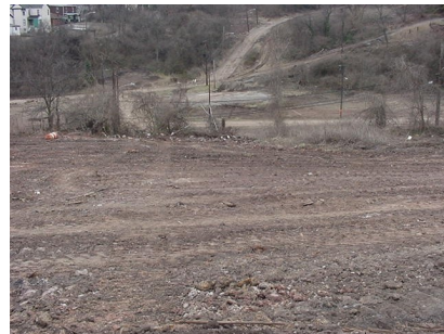
Site After Demo and Rough Grading
